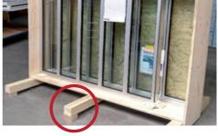
Prior to opening the crate, blocks should be used to lift the base of the crate. The crate must be inclined to the rear at an angle of min.  $4^{\circ}$  to max  $6^{\circ}$ . This prevents the windows from falling out when the transport lock is released. This prevents the windows from falling out when the transport lock is released.
